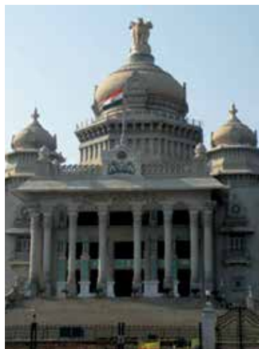
Location: Bangalore, India Project: Hotel Gardenia Application: AB-QM for Heating and Cooling
