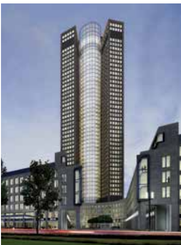
Location: Frankfurt, Germany Project: Tower 185 Application: AB-QM for Heating and Cooling
