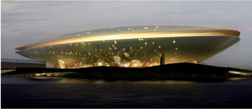
Location: Shanghai, China Project: World Expo Performance Centre Application: AB-QM for Heating and Cooling
