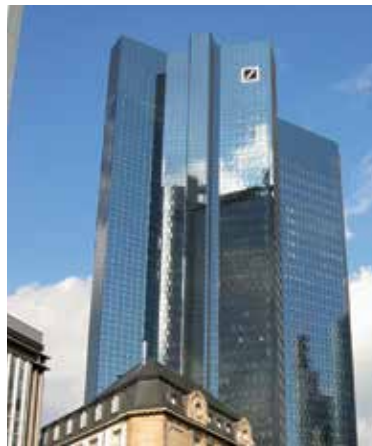
Location: Frankfurt, Germany Project: Deutsche Bank Application: AB-QM for Heating and Cooling
